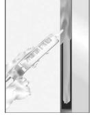
Gun, trowel, or pump approved sealants to minimum 1/4" depth on both sides of wall or top of floor over the backer rod.
