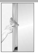
Trowel sealant to the desired finish. See tested UL systems for complete installation instructions.
