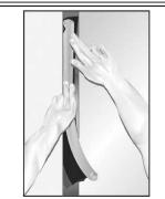
1. Clean all surfaces in joint area to remove loose debris, dirt, oil, wax, grease, old caulking, etc. 2. For floor applications, install a separate base section of backer rod recessed approximately 2" down from the top of the floor. Bend and friction fit Metacaulk<sup>®</sup> Joint Strip longitudinally into joint using the backer rod as the transport mechanism. Push into joint far enough to accommodate the required depth of caulk.
