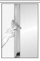
4. Trowel sealant to the desired finish. See tested UL systems for complete installation instructions.
