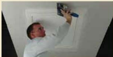
4. Tape and apply drywall compound.
