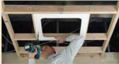
2. Mount Stealth surround with drywall screws.
