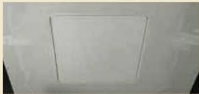
5. Apply desired finish.
